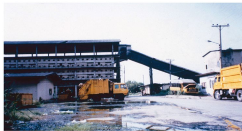
John Thompson composting plant built on the dumpsite around 1960, sold on strength of one operating plant in Jersey (UK) (Breidenbach, 1971). Incoming mixed waste pulverized in a hammermill, then conveyed to top of six-floor building; waste remained on each floor for one day, then released mechanically to next floor down (the aeration process). 'Composted' waste matured for some months before being sieved in a compost finishing plant. Unclear how far the plant had ever been successful; by 1983, still in use but compost no longer sold.
